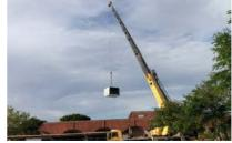
New Air Handling Unit being lifted onto Building 1600
